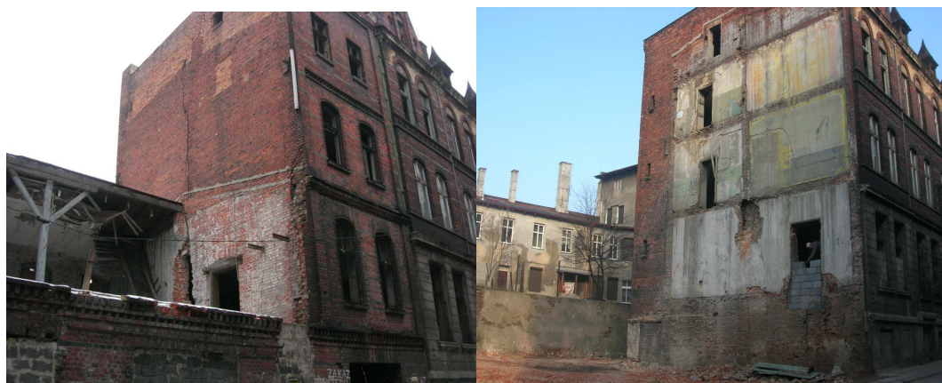
Figure 36. Bytom. Construction disaster at Korfantego Street. Just before and just after
