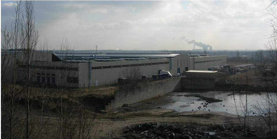
Figure 8. Sosnowiec. New investments localised on brownfields in The Katowice Special Economic Zone. The Investment Area “Dańdówka”
