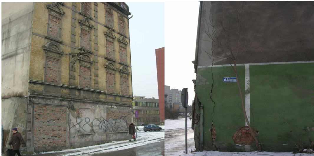
Figure 38. Bytom-Rozbark. The mining damages effects on pictures from the winter of 2010. Tilting building (on left) as well as cracked walls in other (on right). Building on left picture has been demolished finally in 2011
