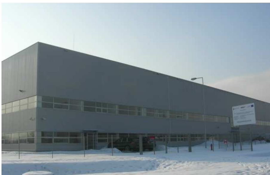
Figure 43. Sosnowiec. “Watt” Company localised in the investment area “Mikołajczyka” of the KSEZ
