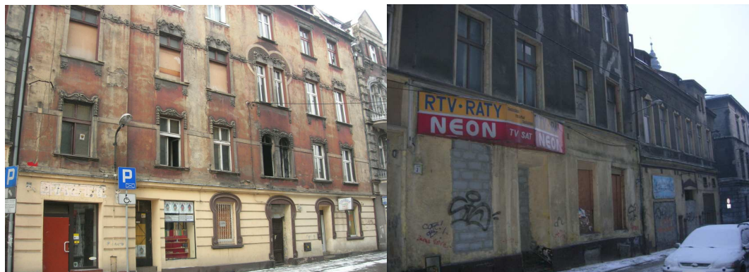
Figure 34. Bytom. Abandoned flats and shops in city centre
