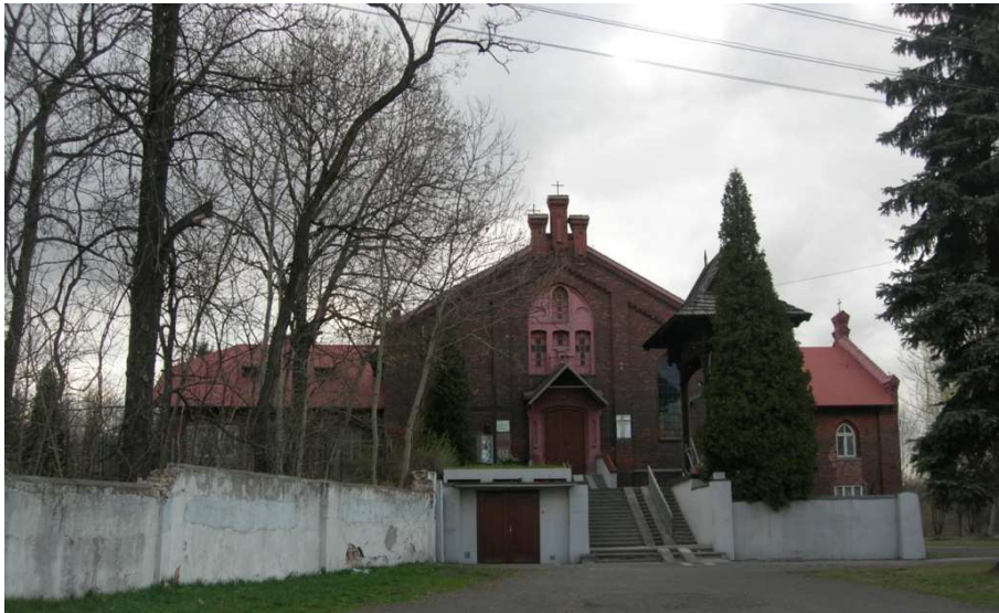
Figure 25. Sosnowiec-Porąbka. Former post-mining building conversed into a Catholic church
