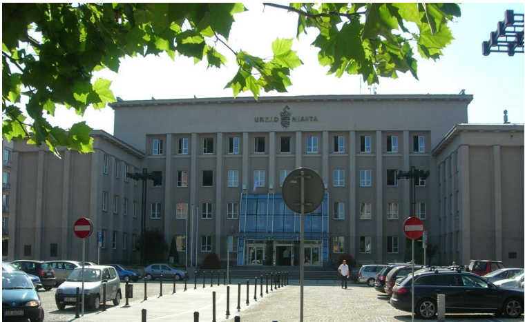
Figure 7. Municipal office in Sosnowiec
