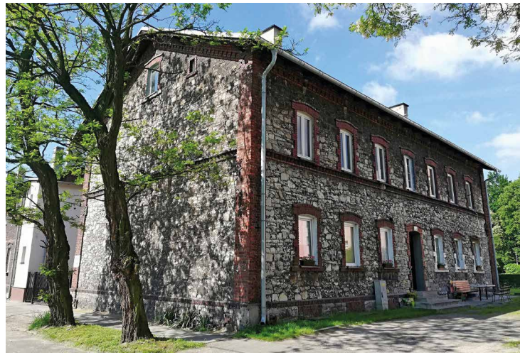
Company-sponsored housing estate in Czeladź, Piaski district
