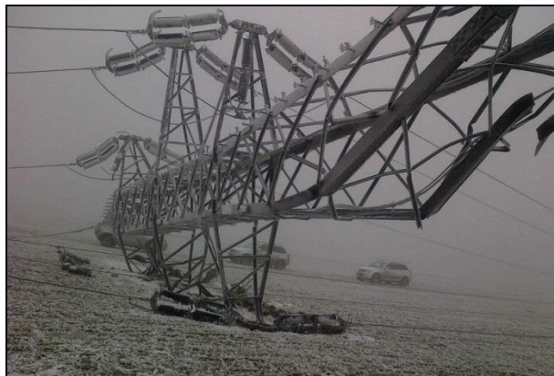
Figure 4. High-voltage masts collapsed due to icing
